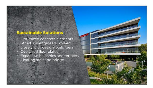
The structural engineers worked closely with the design-build team to meet a demanding schedule, structural challenges, and environmental criteria for this concrete building. The design required oversized floor plates to accommodate open office spaces, expansive balconies and terraces, and large meeting spaces. They also made the designer's vision for a truly unique lobby space come to life with a floating stair and bridge that lead visitors to large meeting spaces.
