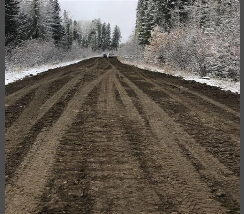
Reapply the aggregate taken from the road. Final product is stable with excellent drainage.
