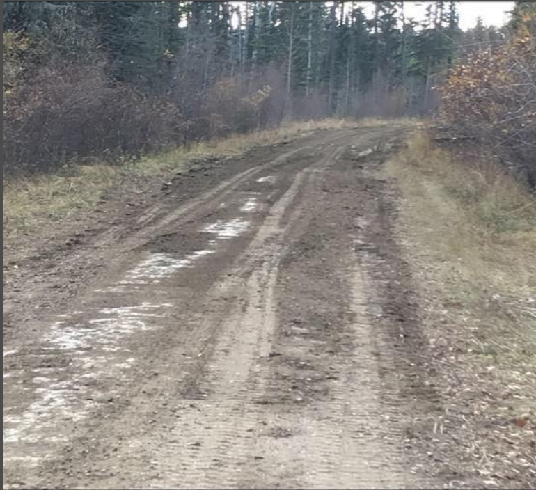
Existing road has soft shoulder issues and pooling water and mud where vehicles become bogged down.
