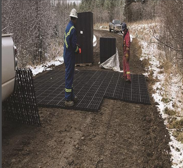
Top layer of the road is removed and grid is applied.
