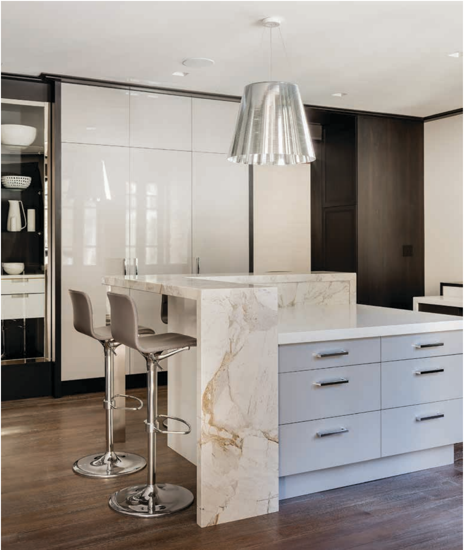
"The undersides of both islands are exposed at the seating areas," explained John Kilfoyle of United Marble Fabricators in Watertown, MA. "These areas are also mitered and fully polished underneath so that no visible area is dissimilar."
